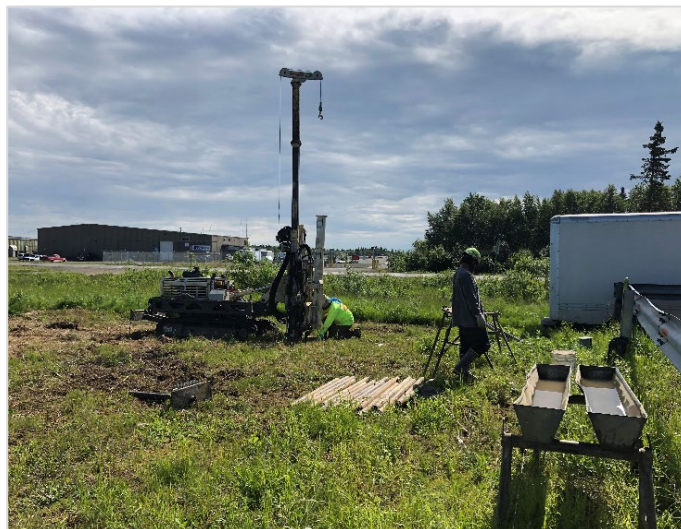
Exhibit 4-1: Drilling near long-term airport parking
