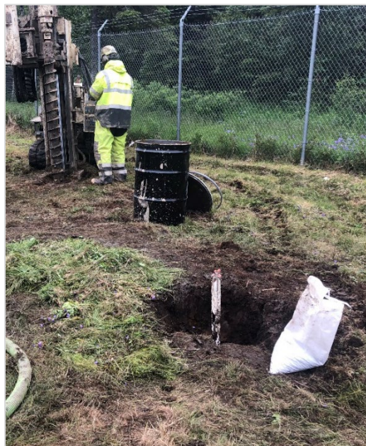
Exhibit 2-3: Well installation at MW03
