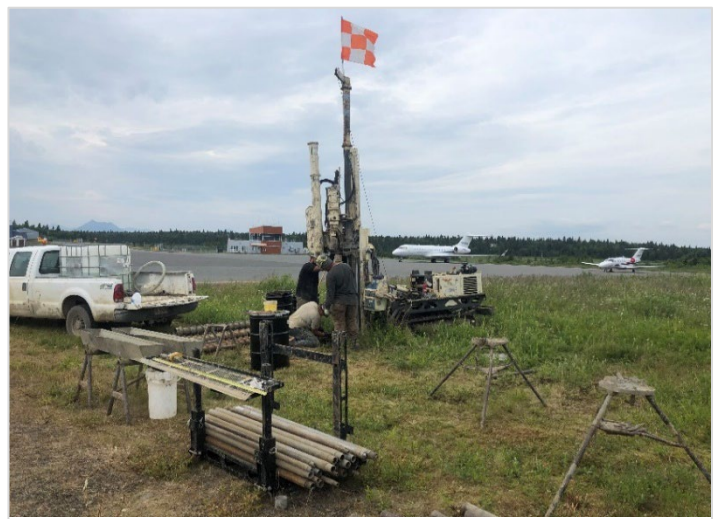
Exhibit 2-2: Drilling near the Taxiway B windsock
